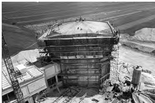
The Reactor Centre, Podgorica, built in 1966
