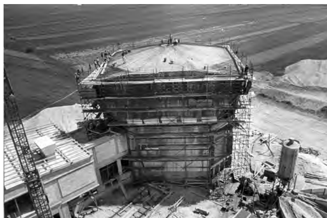
The Reactor Centre, Podgorica, built in 1966
