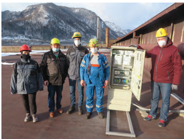
Figure 3: Solar potential test field on the roof of SIJ-Acroni plant (project CREATORS).
