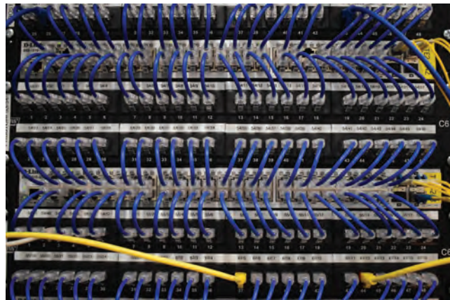
Figure 4: Modern cabling with custom patching cables allow us to deliver clean, easy to maintain network set-ups, as seen in this network cabinet at Teslova.
