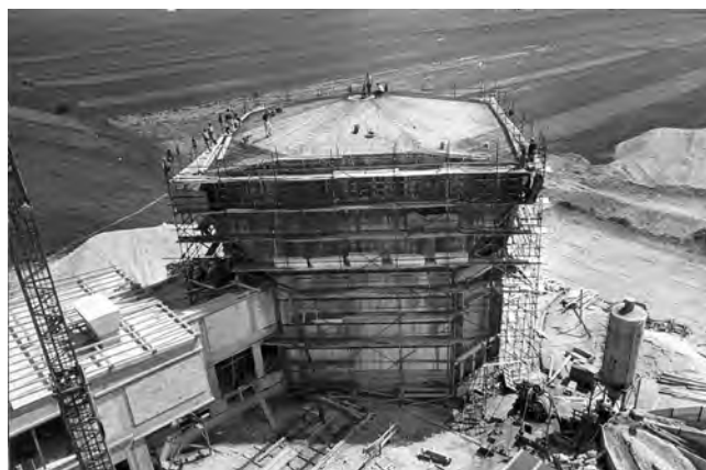
The Reactor Centre, Podgorica, built in 1966
