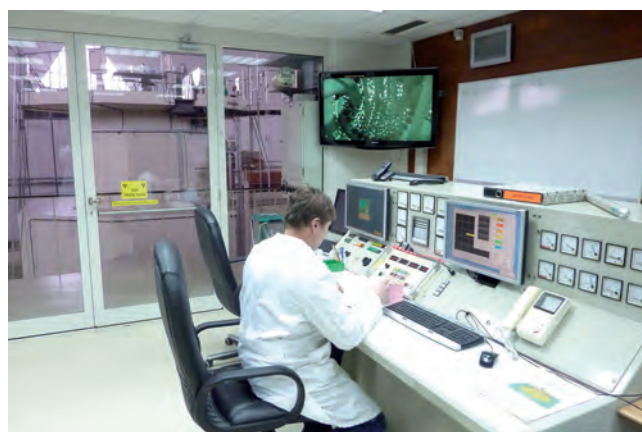
Figure 1: Renovated control room of the TRIGA reactor
