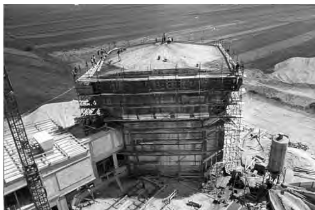
The Reactor Centre, Podgorica, built in 1966
